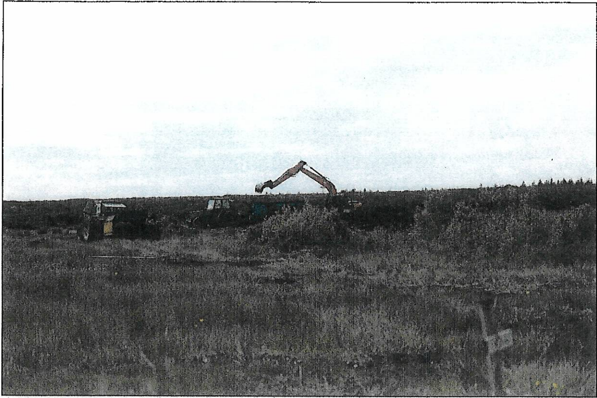
Figure 5: EVIDENCE OF POTENTIAL UNAUTHORISED ACTIVITY 07/06/21
